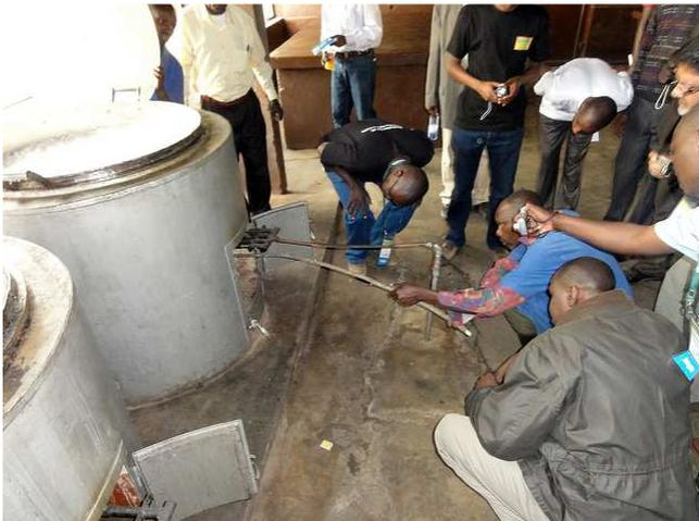
Figure 6: A stove in a school kitchen running on biogas produced from human excreta in Rilima, Rwanda (source: P. Feiereisen, 2011). More photos on this school: [www.flickr.com/photos/utzecosan/sets/72157627230220319/with/6008002835/](http://www.flickr.com/photos/utzecosan/sets/72157627230220319/with/6008002835/).
